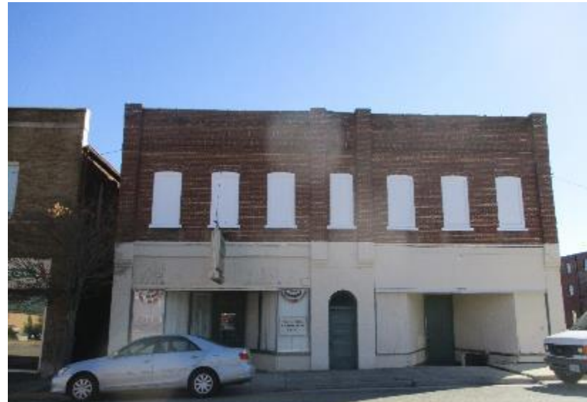
Photograph 34: Historic doors on secondary entrances should be retained.
