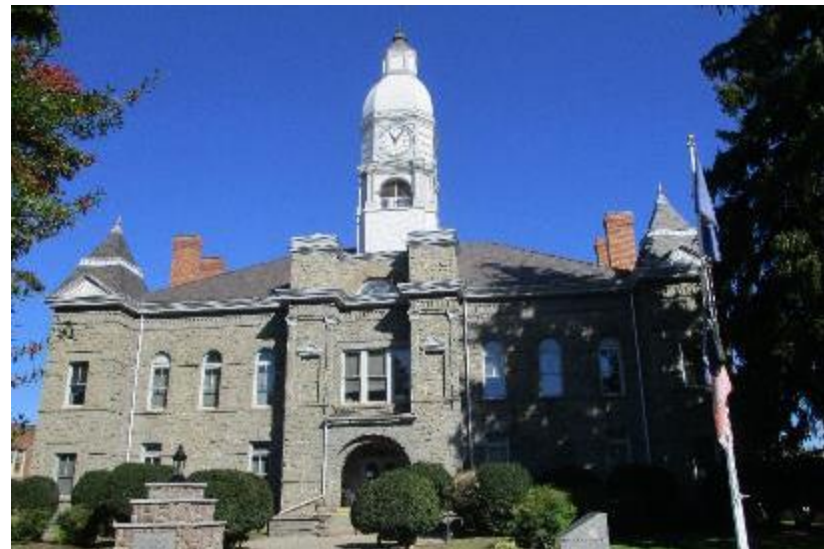
Photograph 11: Example of a Romanesque Revival/Richardsonian building.
