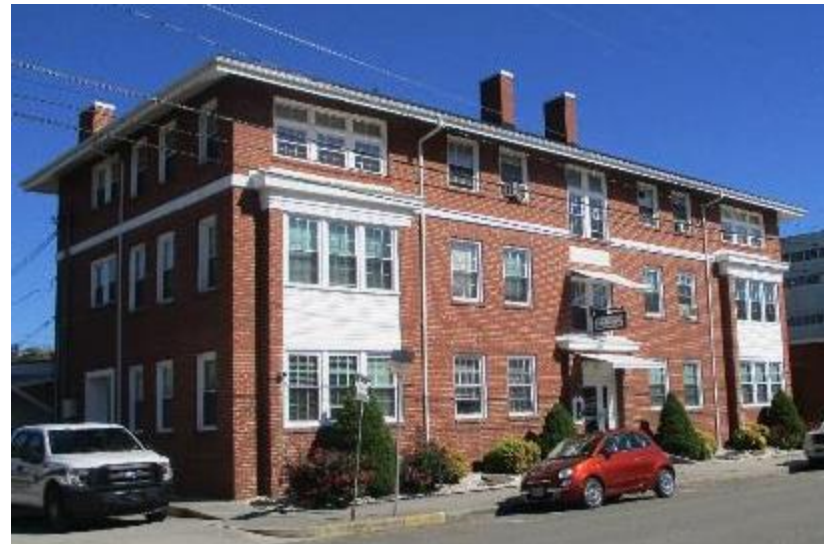
Photograph 17: This apartment building has Craftsman style influence.
