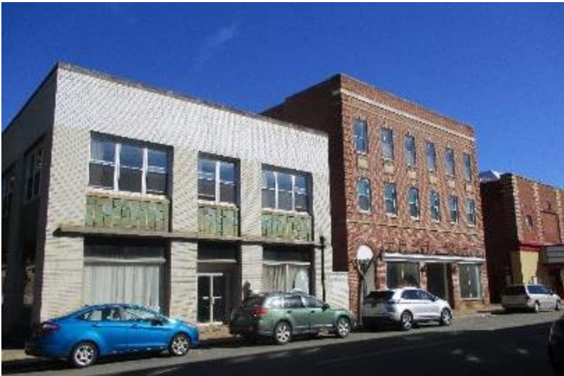
Photograph 6: View of historic district along Main Street.
