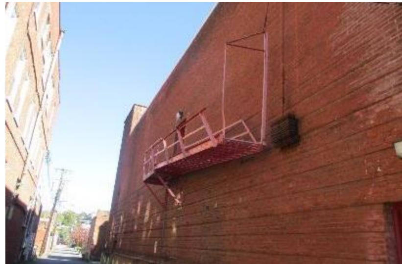
Photograph 43: Fire escapes and exterior stairs should be placed on non-visible elevations wherever possible.
