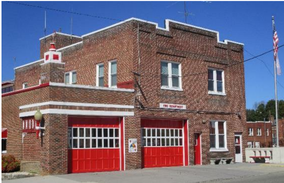
Photograph 21: Regular maintenance is the best conservator of any historic building.
