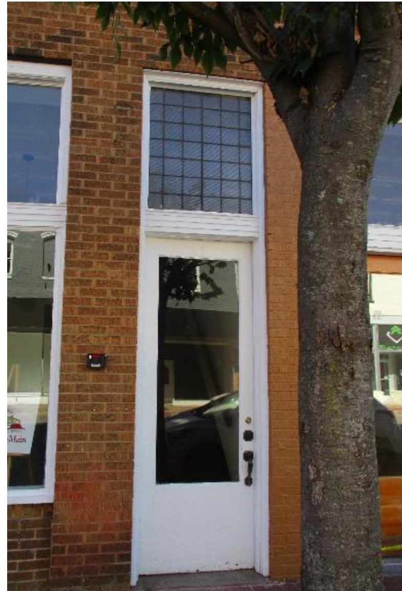
Photograph 36: Transoms and door surround should be retained.
