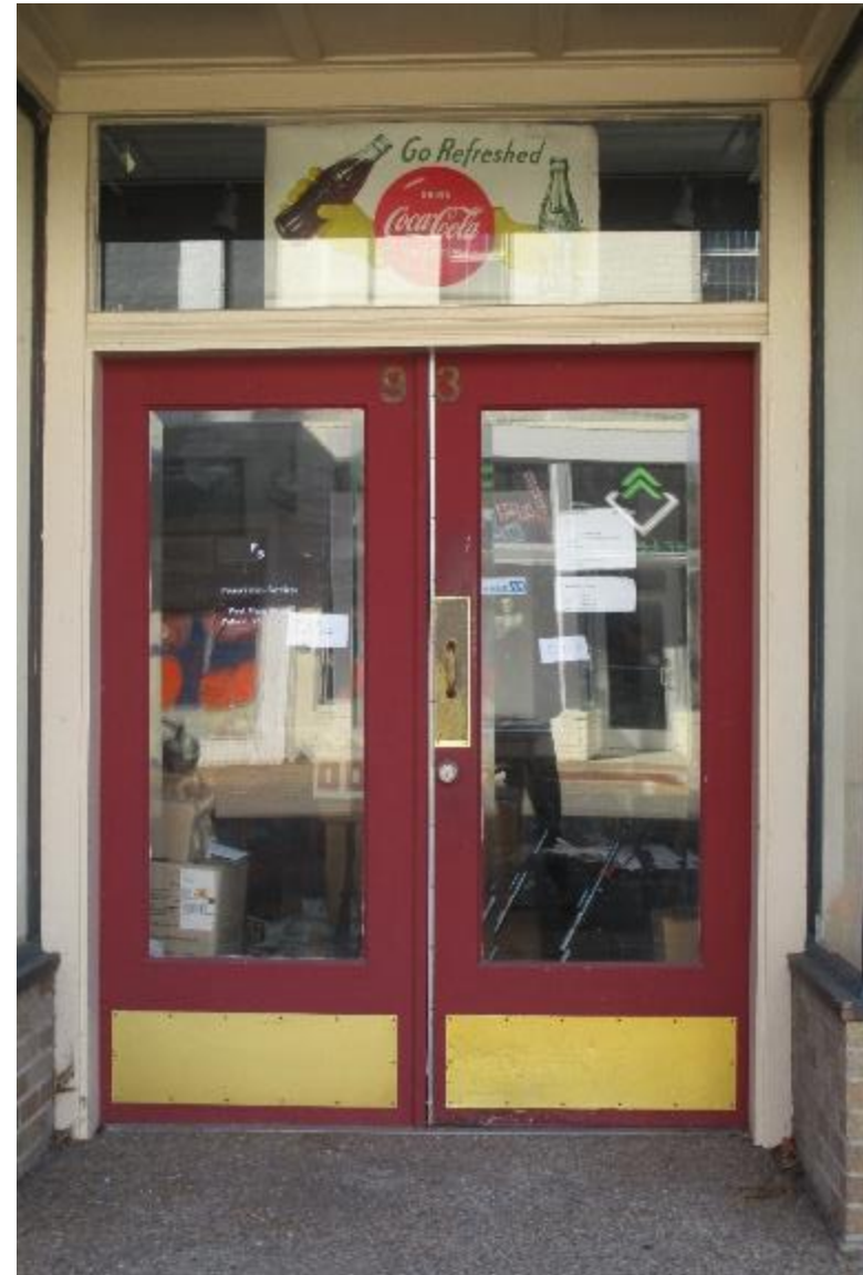
Photograph 39: Painted elements should typically remain painted.
