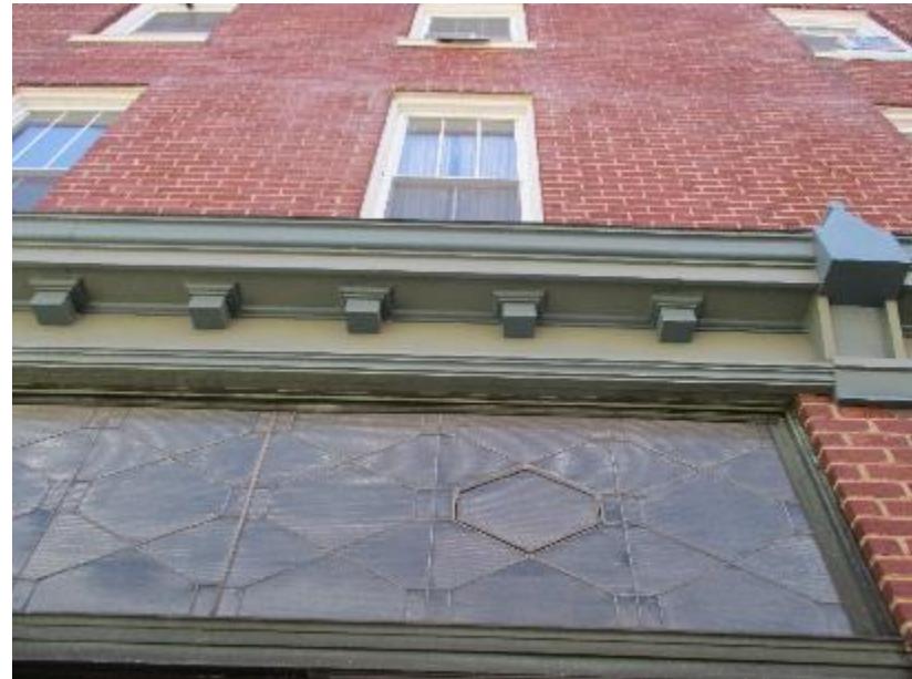
Photograph 33: Historic transoms and original window sashes should be retained where present.
