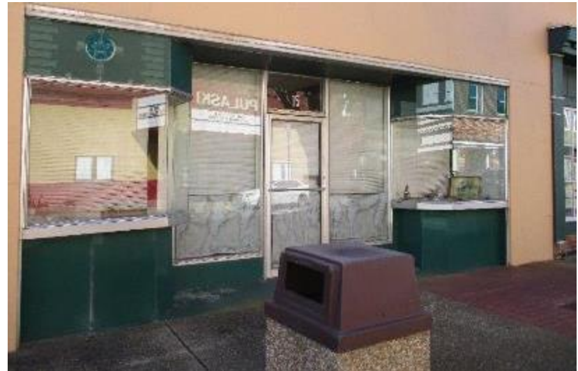
Photograph 28: A storefront with Art Deco influence. Storefronts with architectural significance should be retained.
