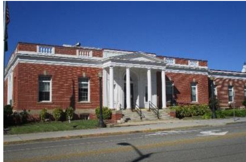
Photograph 16: The US Post Office is an example of Colonial Revival style building.
