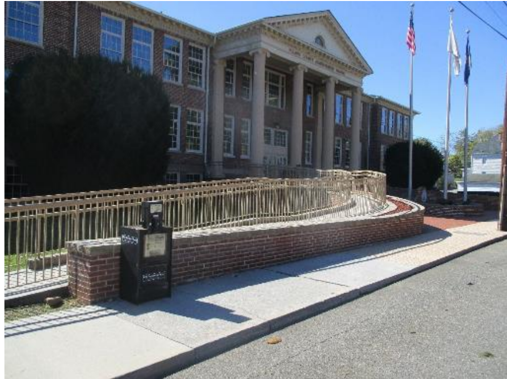
Photograph 41: ADA ramp designs should be inconspicuous or integrated with the building's architecture.
