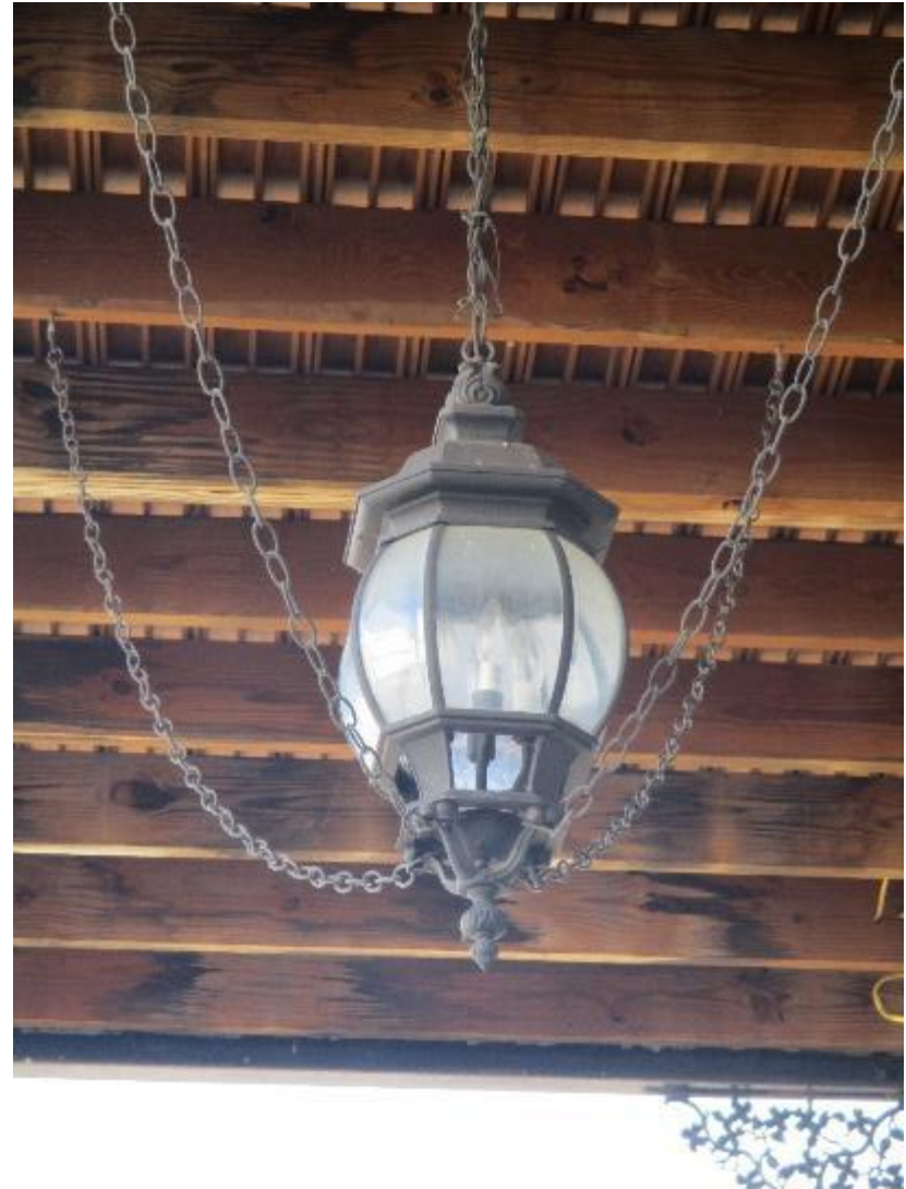
Photograph 44: Exterior lighting should be appropriate to the building's character.
