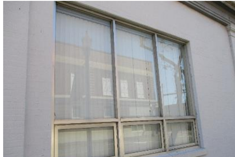
Photograph 30: View of aluminum windows on a commercial building.
