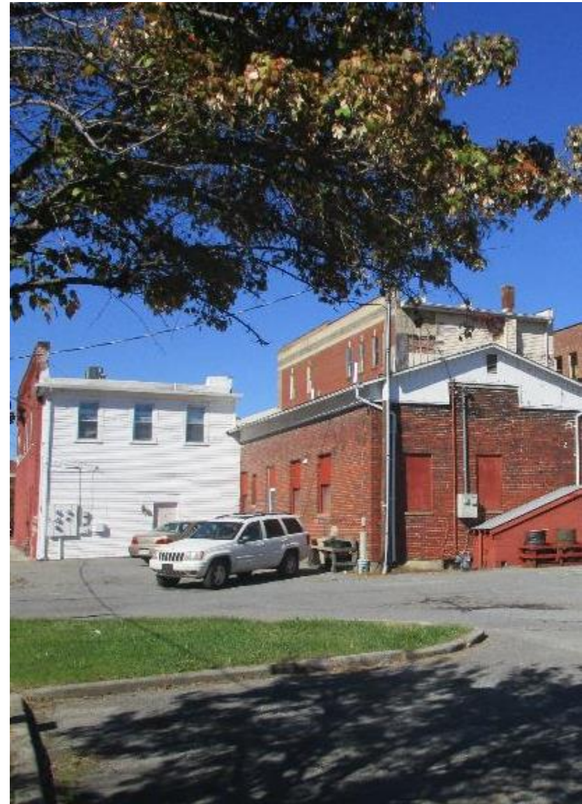
Photograph 26: Most buildings in the Commercial Historic District do not have siding but it may be appropriate for side elevations.
