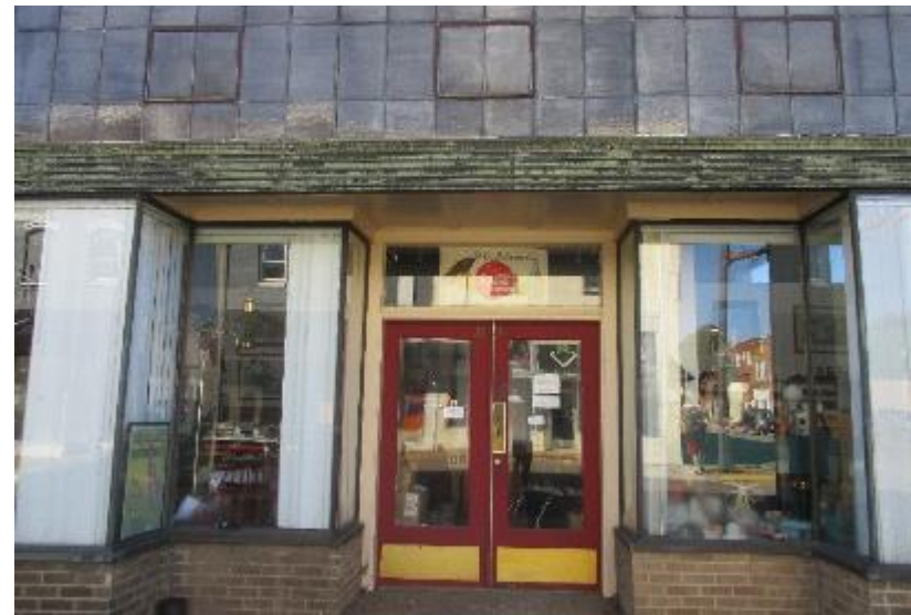
Photograph 35: Existing historic doors should be retained and restored where possible.
