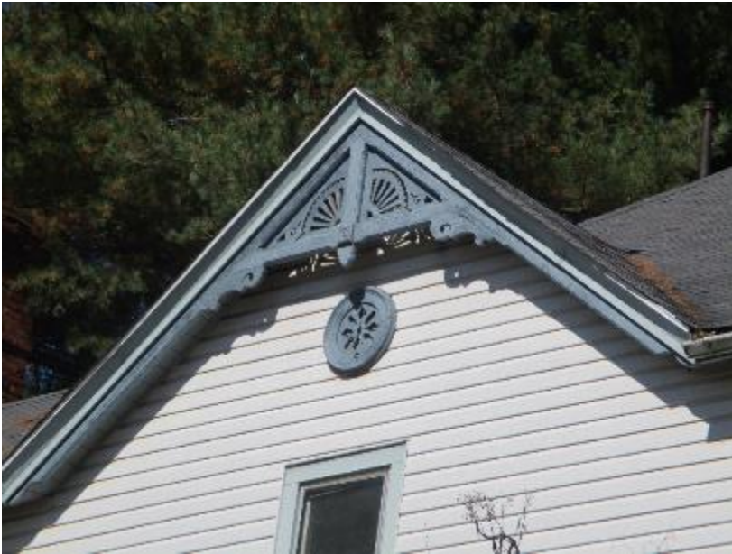
Photograph 37: Decorative woodwork should be retained where present.
