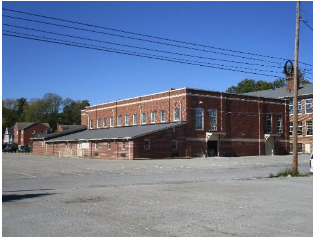
Photograph 40: This historic addition is not a character defining feature, however, it does not compete with the original historic building or the surrounding district.
