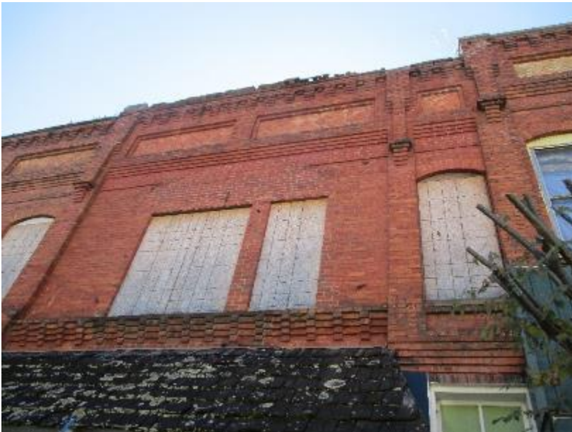
Photograph 32: Historic window openings should be retained.
