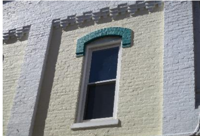
Photograph 31: View of double-hung windows on the residential portion of a commercial building.
