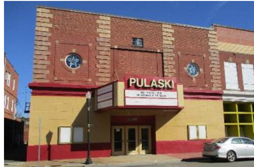
Photograph 18: The Pulaski Theater's sign and lower stories have Art Deco details.
