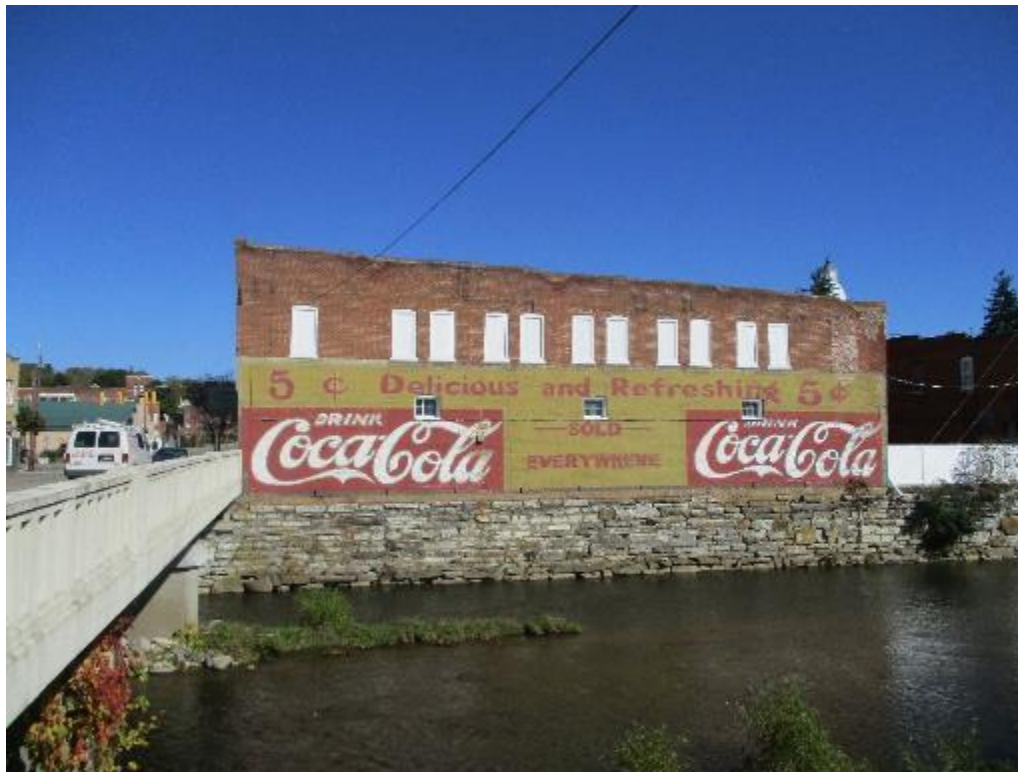
Photograph 52: Historic wall signs should be preserved, however, painting previously unpainted brick should be avoided.
